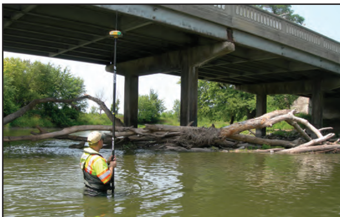
Graduate student Richard Liggett collected bathymetric data in the Big Sioux River near a bridge outside Flandreau, SD. Field survey data are entered into computer models to predict flow characteristics and the associated bridge scour depths produced by large floods.
