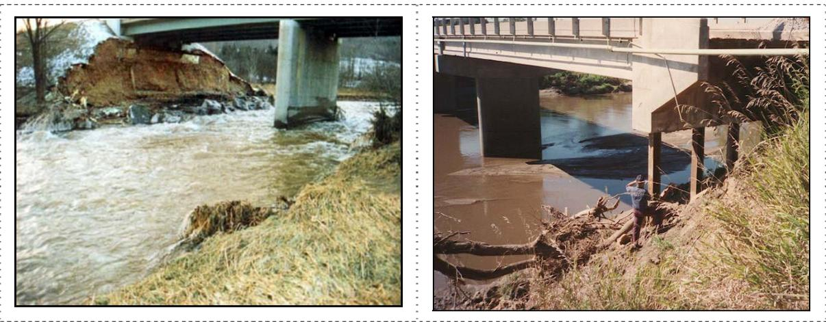
*Figure 1. Abutment failure due to scour typically is attributable to the geotechnical failure of the abutments spill-slope, as illustrated by these two examples.*
