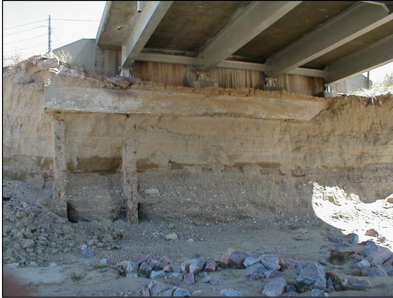
*Figure A-3. View of an eroded spill-slope bridge abutment at bridge at Cottonwood Creek, WY. Abutment scour eroded the channel bed, which then resulted in spill-slope failure (including collapse of riprap rock). Lateral erosion of exposed spill-slope soil ensued (Photo courtesy of William Bailey, WYDOT)*
