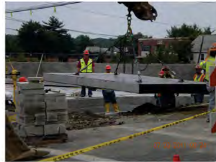
Precast Approach Slab Installation http://www.flickr.com/photos/25664139@N00/5899098381/ Accessed 16 Nov 2012
