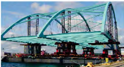
Replacement of Truss Span without Deck (Barge Use) http://www.ftwa.dot.gov/bridge/abc/docs/aashto.pdf Accessed 23 Oct 2012
