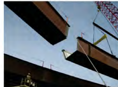
Steel Tub Girder Placement http://www.highsteel.com/project_gallery/bridges/Brightman-Street-Bridge.cfm Accessed 23 Oct 2012
