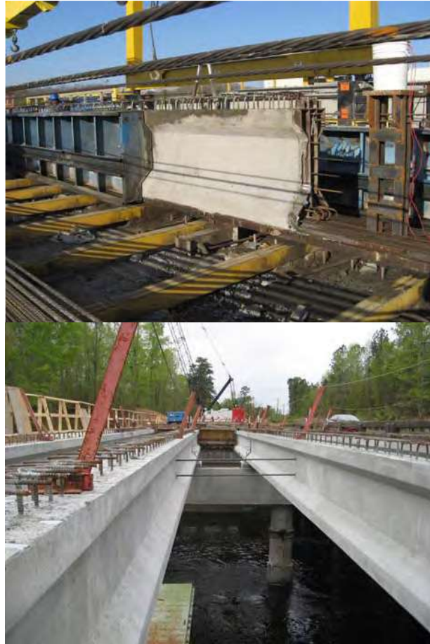
Figure 2 Use of Prestressed SSC Bridge Girders at SCDOT [Error! Reference source not found.].
