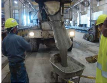
a) SCC Placing
