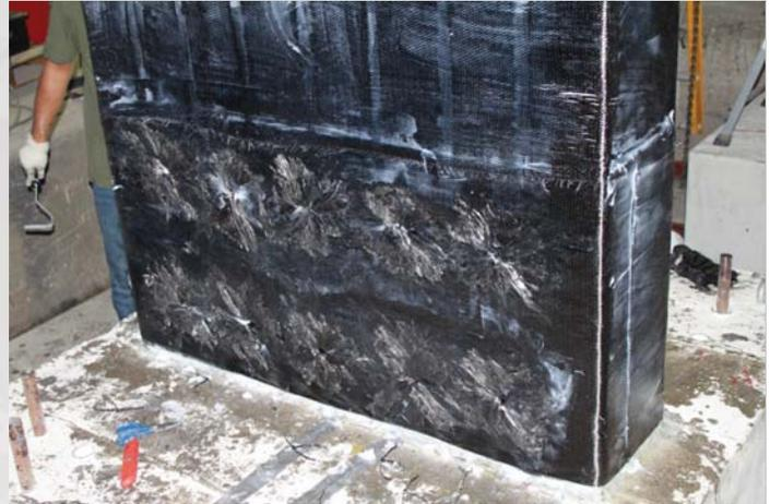
Transverse (horizontal) CFRP anchors
