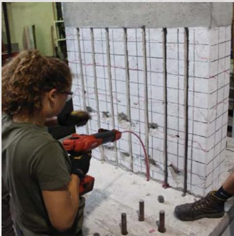
Mild Steel NSM bar placement
