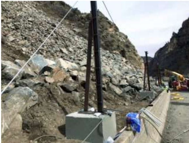
Figure 1. Construction of rockfall barriers along I-70 in Glenwood Canyon. The individual boulders in the background have the potential to be individually imaged and cataloged to monitor their changes in position as a function of time to estimate threat levels to the adjacent highway.
