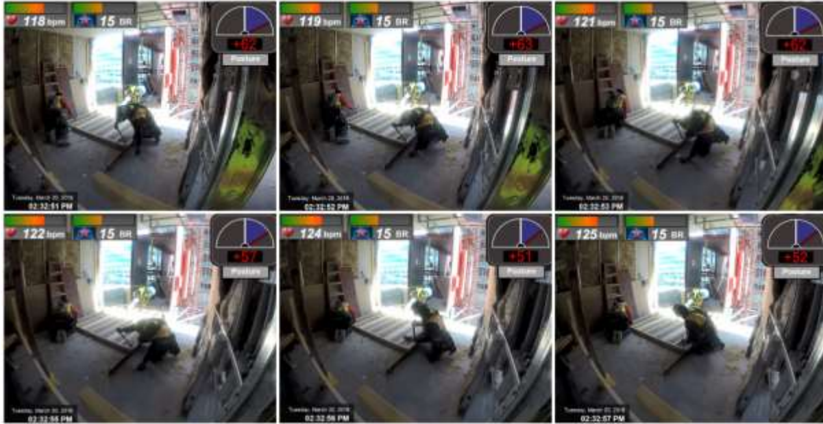
Figure 3: Sample time-stamp series of video feed showing synchronous display of construction worker physiological data and activity.
