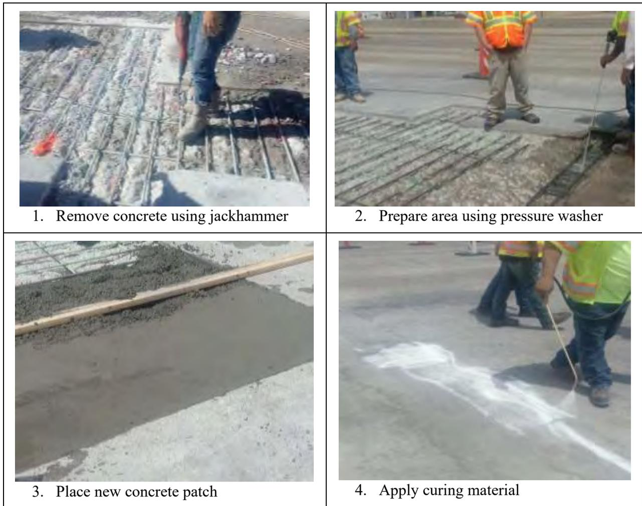
Figure 1: Construction steps of partial-depth repair for concrete bridge deck
