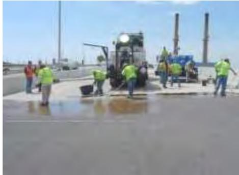
**Figure 1 Overlaying concrete bridge deck with polymer concrete [9]**
