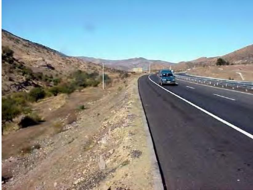
Figure 1. A Rural Roadway with Severe Side Slope
