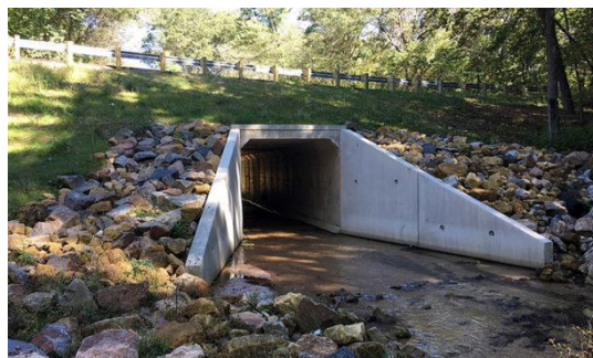
Figure 1. Culvert under a road
